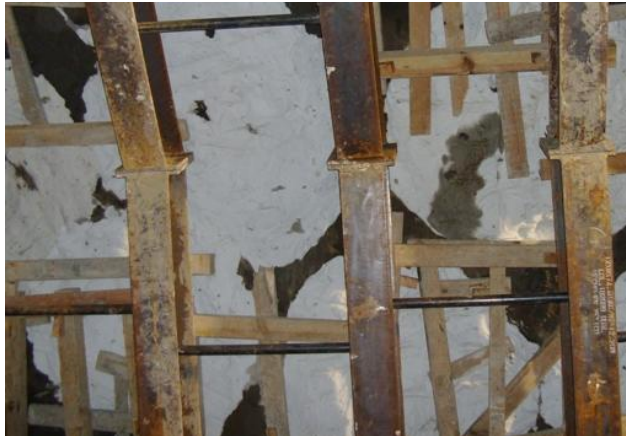
Figure 9. Jet Grouting columns in tunnel code. The metallic frames formed by an IPR section of 12x8" (74 kg/m), ASTM A36, separated every 2.0 m can be seen
