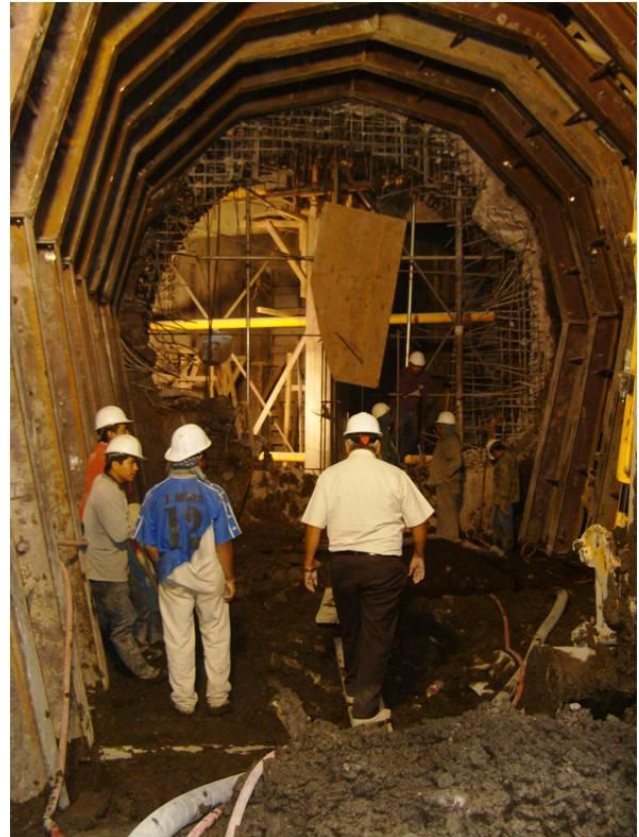
Figure 10. Excavation of one of the interconnection tunnels, with conventional procedure. The metallic frames placed for the excavation's safety stand out
