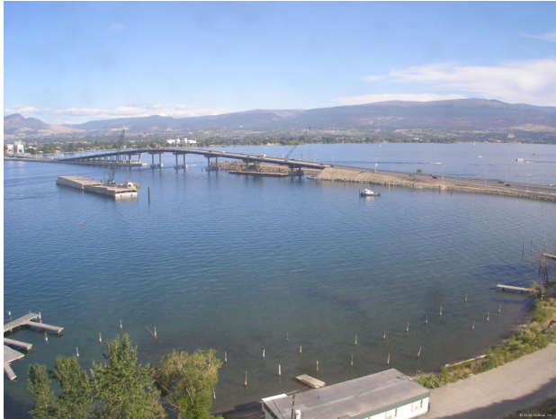
Figure 2. Photograph showing the bridge crossing
