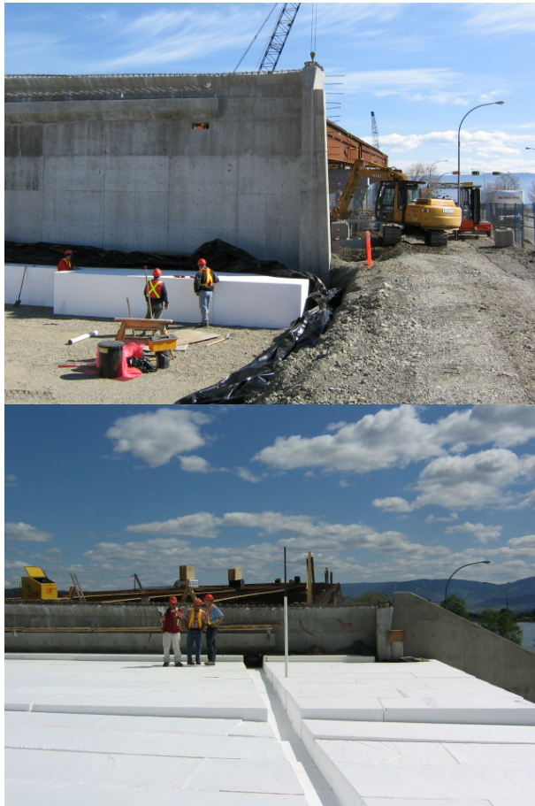
Figure 11. Photographs showing placement of EPS fill
