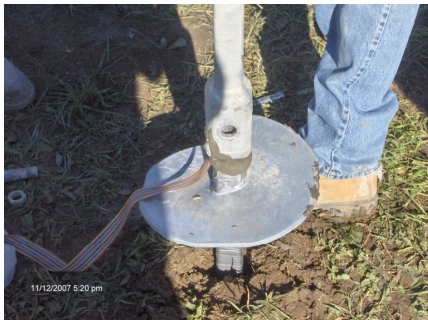
Figure.5.a. Typical preparation of lead section – extension connection
