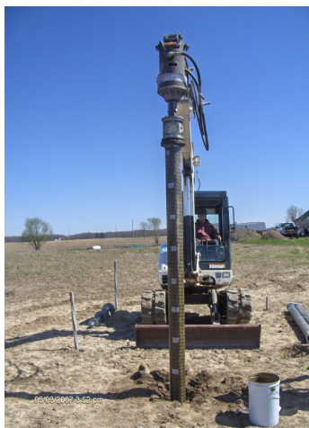
Figure. 5.b. FRP-G-HSP installation (internal SS175 shaft – external FRP 3m tube).
