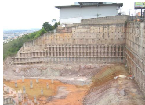
Figure 1. Anchored wall and building behind.
