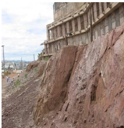
Figure 2. Bottom of the anchored wall where 70^\circ discontinuities can be seen.
