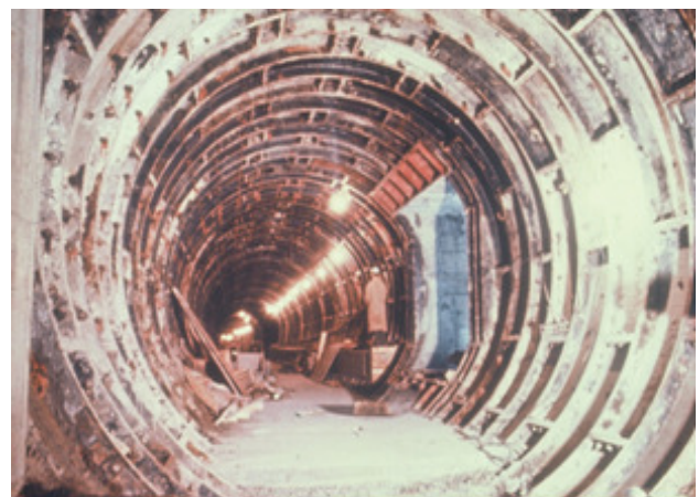
Figure 2. TTC Subway tunnel
