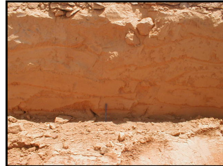
Figure 3. Excavation in collapsible soils showing vertical walls and big lumps of soil.
