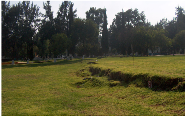
Figure 7. Soil fracture in transition zone (LGI, 2008).
