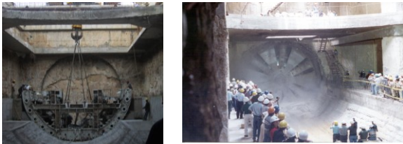
Figure 11. Subway construction in Valencia, Venezuela
