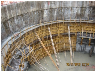
Figure 13. Shaft excavation for sewer pipeline in Panama
