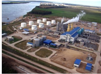
Figure 12. Timbues Power Plant in Santa Fe, Argentina.
