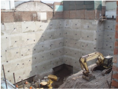
Figure 10. Seven level basement excavation in Lima, Perú.
