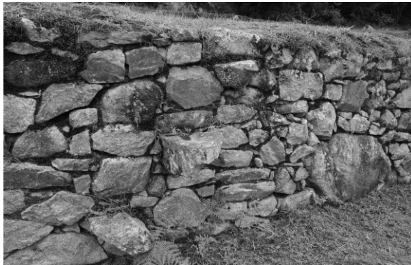
Figure 2. Photograph of the Inca wall selected for the stability analysis
