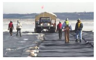
Figure 1. Preparing to sew a seam on the ice. Note stockpile of coke in the background.
