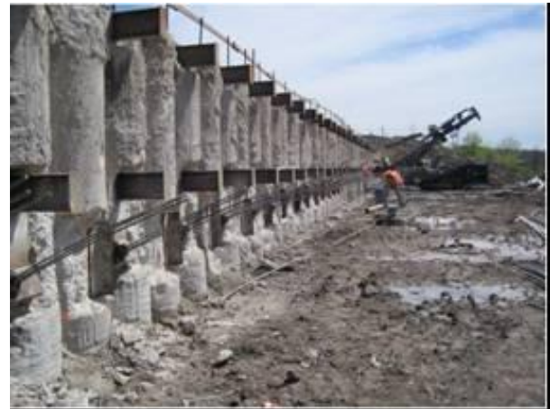
Photo 1. Caisson wall supported by tiebacks at Waterloo WWTP
