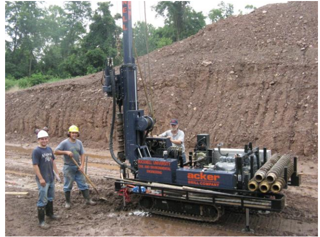
Figure 2 Drilling rig used for cutoff wall testing
