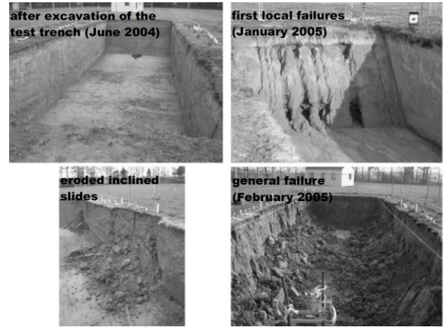
Figure 6. Field tests on the stability of trench in an unsaturated soil deposit (Whenham et al. 2007).
