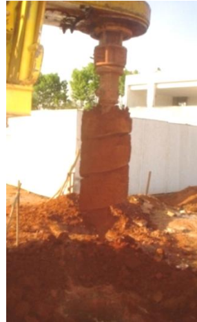
Figure 7. Column borehole execution.
