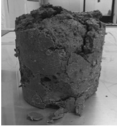
Figure 2- Degradation of a specimen after 7 f/t cycles
