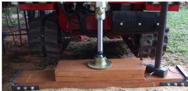
Figure 6. Bigger shear beam placed in the rear of the pushing equipment.
