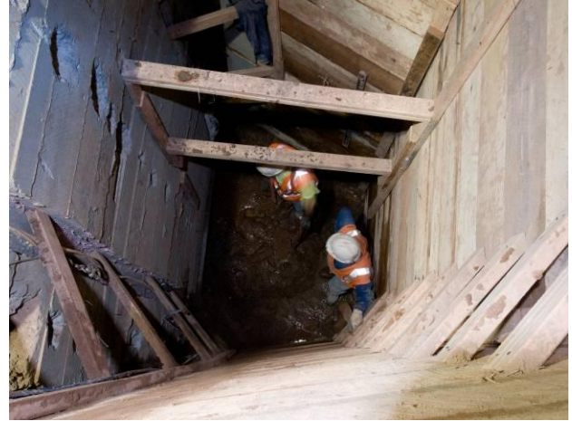
Figure 9. Hand excavated pit.
