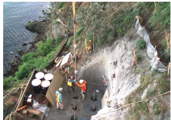
Figure 5. Micropile construction at A1
