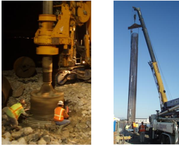
Figure 9. Drilling and rebar cage installation at Tower C CIDH pile
