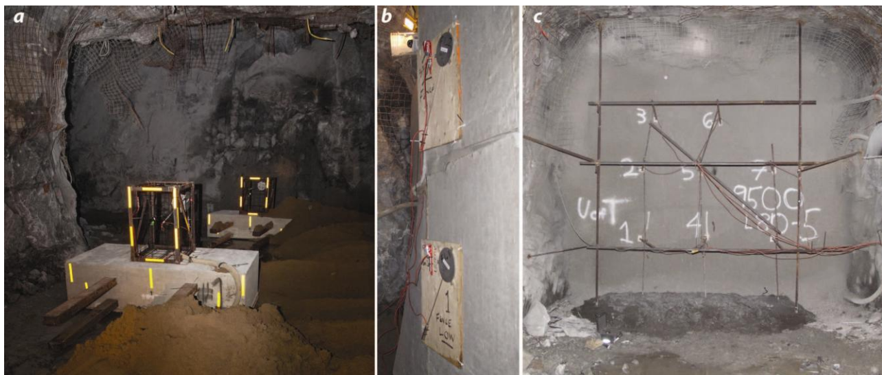
Figure 7. (a) Cages in undercut of stope. (b) TEPCs and piezos on barricade. (c) Barricade displacement array
