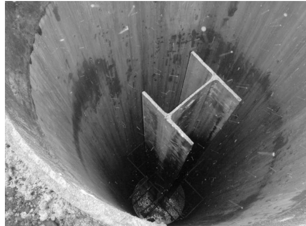
Figure 6. Pile with Steel Beam Profile
