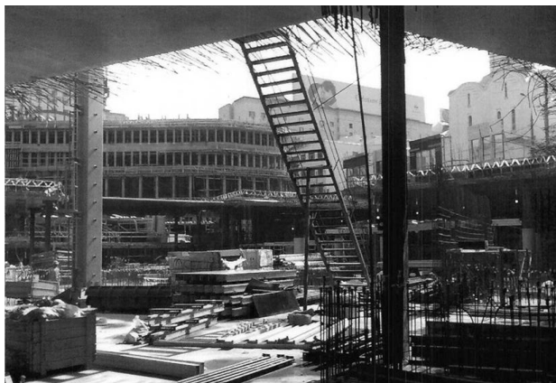
Figure 9. View from under beneath the ring slab.
