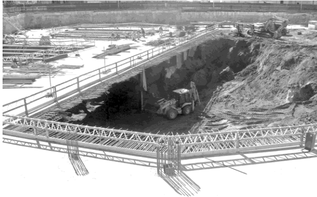
Figure 8. Excavation under the ring slab.
