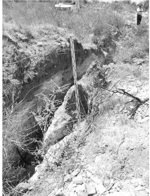
Figure 11.- Surface fault related to differential sinking in the Aguascalientes City.
