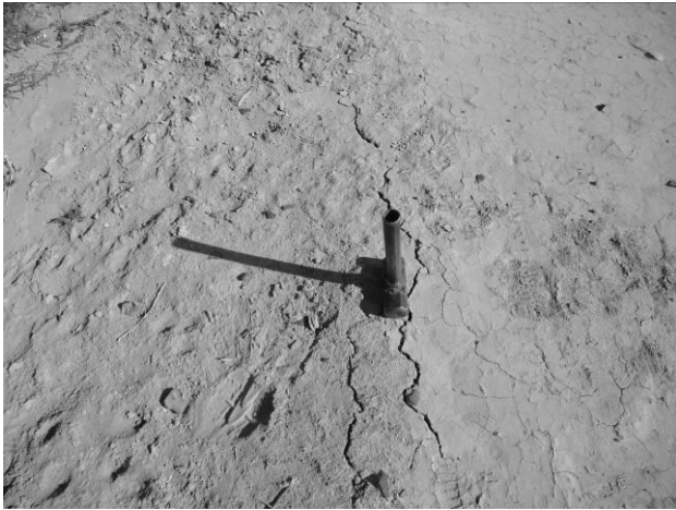
Figure 15. Soil crack in a first stage of formation
