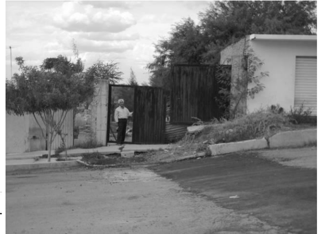
Figure 3. Ramp developed by a soil crack at the northwest of the City of Aguascalientes. The vertical displacement of the blocks generated by the rupture is evidenced by the gate.
