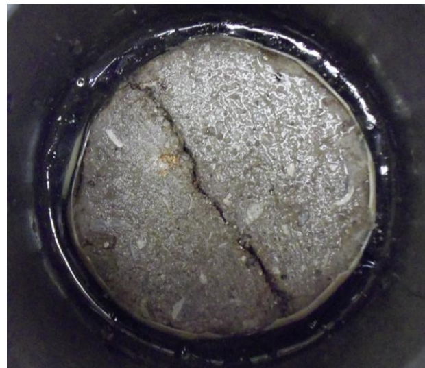
Figure 4. Cracked SCB core for laboratory permeability testing.
