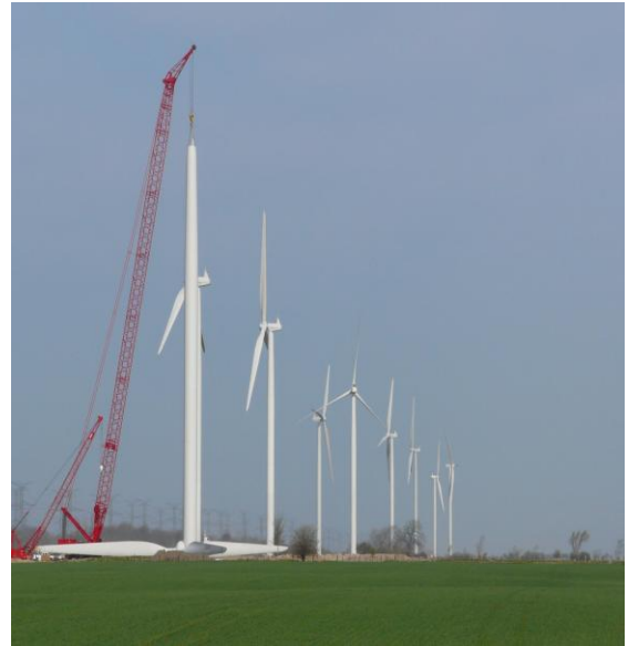
Photograph 1. Example of Wind Turbine Erection
