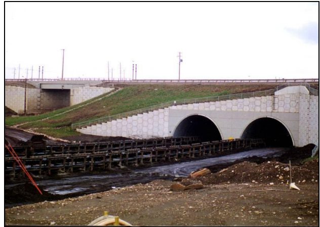
Figure 9 Foreground Arches over Conveyors, Background MSE Bridge over Haul Road
