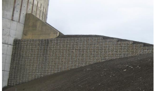
Figure 5 Wire Faced Wall with Gabion Rock
