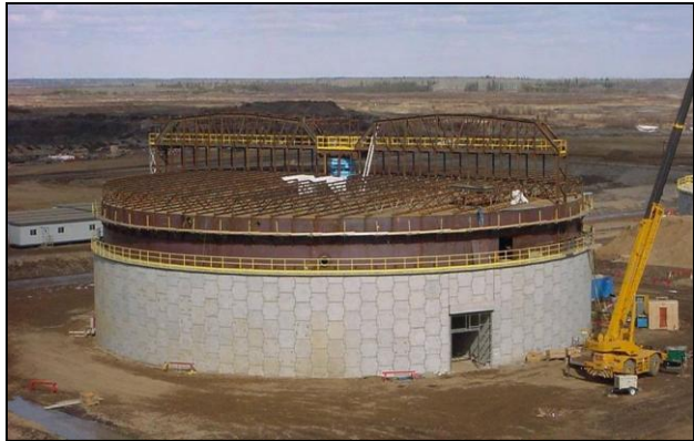
Figure 16 Completed Froth Settler Tank
