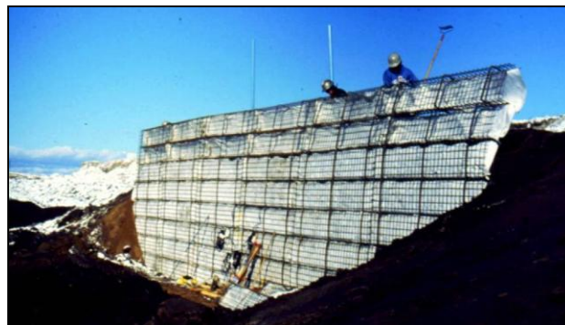
Figure 8 Lean Oil Sand Test Structure
