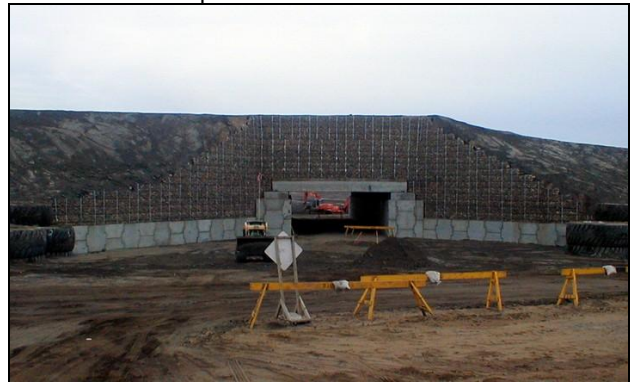
Figure 10 Bridge to Carry Haul Road over Conveyors
