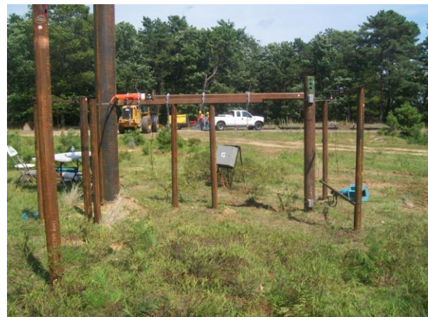
Figure 3. Typical lateral load test setup
