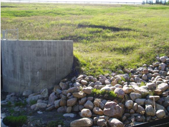
Figure 1. General view of the south slump.
