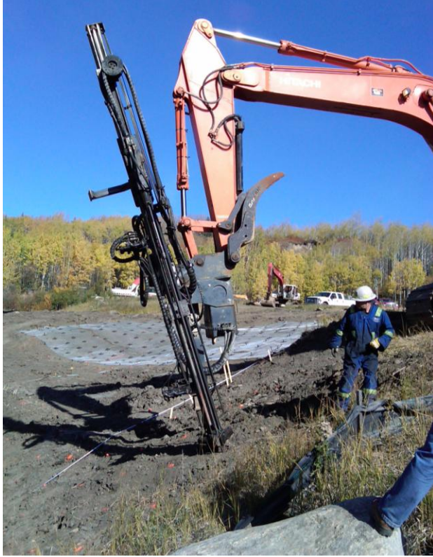
Figure 5. Percussion soil nail installation equipment.
