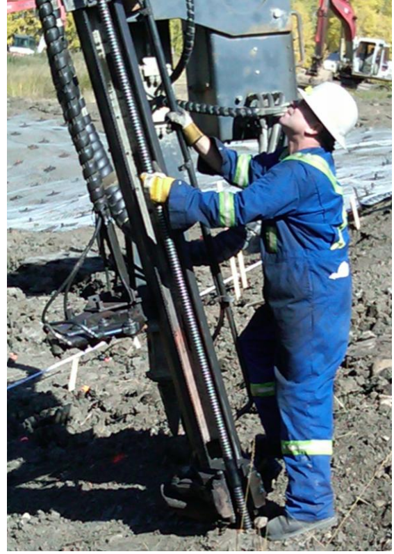
Figure 6. Splicing the second 3 m segment of the nail.
