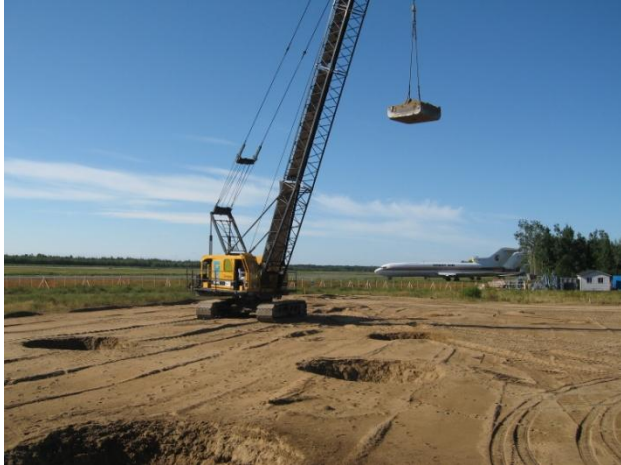
Figure 9. DC crane working away from the building.
