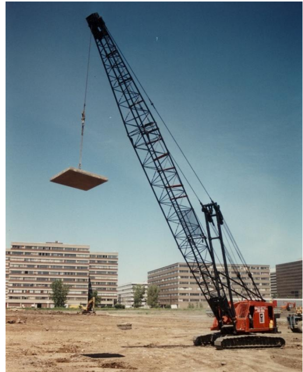
Figure 3. Crane lifting an ironing 10 tonne tamper
