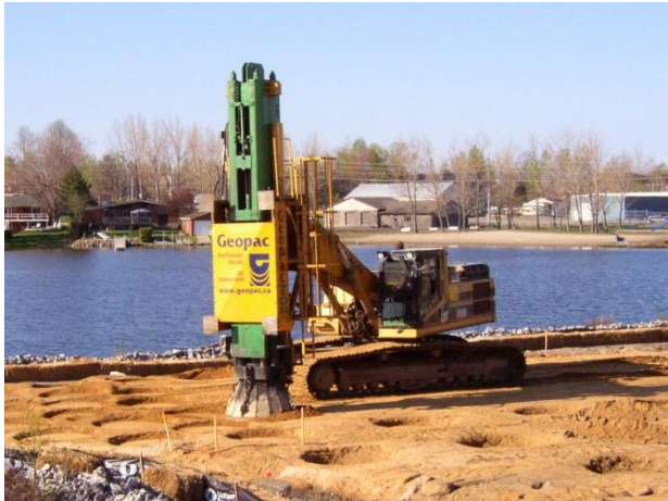
Figure 4. Geopactor RIC rig at work in North Bay (Ontario).
