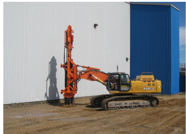
Figure 8. RIC rig working close to the existing hangar.
