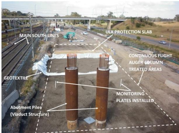
Figure 13. Construction of CFA columns/LTM system under progress
