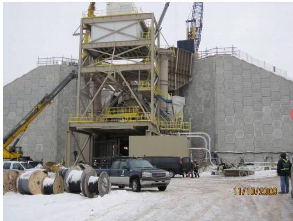
Figure 15. MSE Wall installation complete
