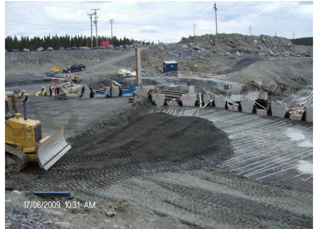
Figure 11. During construction of this Project (long strips and wide area of compaction)
