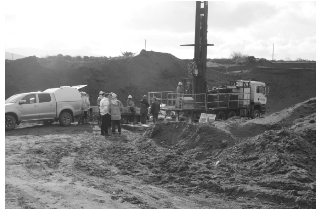
Figure 3: Sonic Coring at Blessington Sand Quarry
