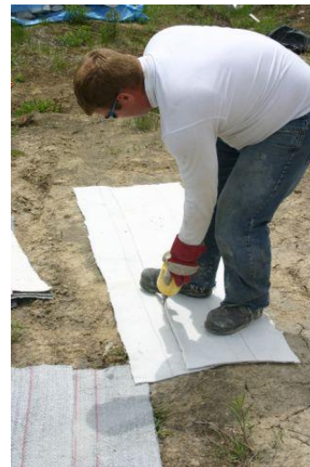
Figure 3. Heat-tacking GCL panels to form a seam.
