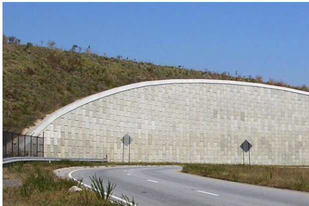
Figure 1 – view of an MSE Wall structure
