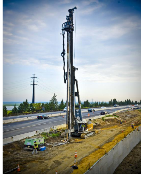
Figure 8 – View of CMC installation during construction of the MSE Wall
