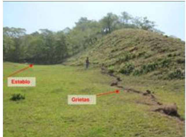
Figure 7. Detail of cracks on the hill adjacent to Cut XV. INGETEC (2009)
