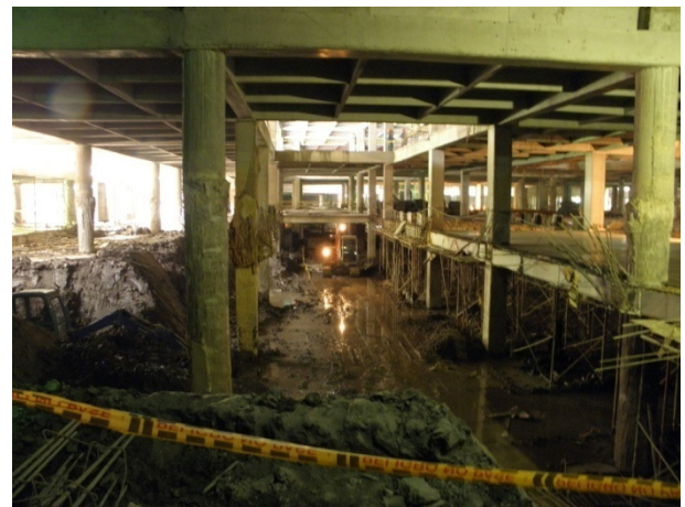
Figure 5.5 Construction of mat under first floor slab.
