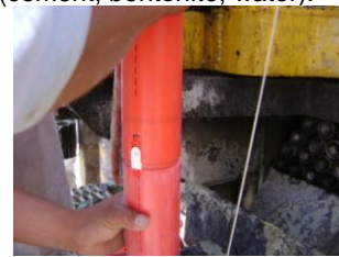
Figure 4. Installation of inclinometer casing.
