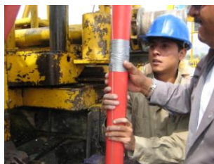
Figure 6. Maneuvers required to install the inclinometer casing
