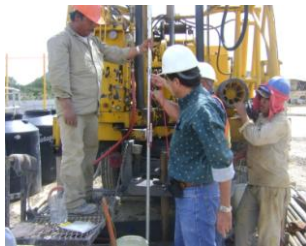
Figure 11. Installation of vibrating wire piezometers
