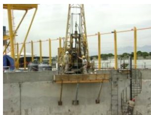
Figure 7. Working platform to install the inclinometers through the diaphragm wall
