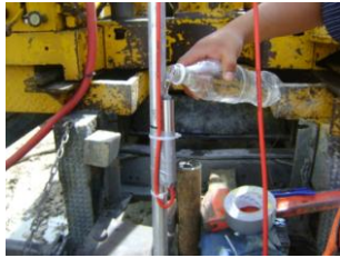
Figure 10. Saturation of piezometers prior to their installation
