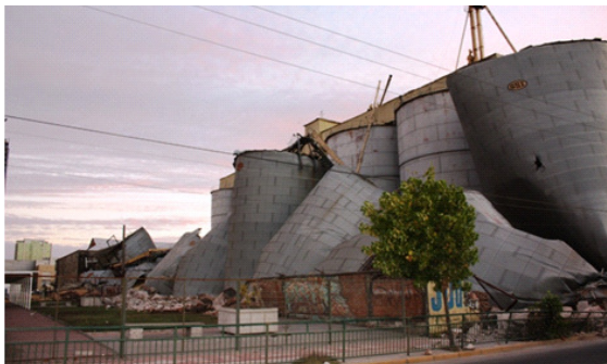
Figure 2. Silos that failed at center of Concepción.
