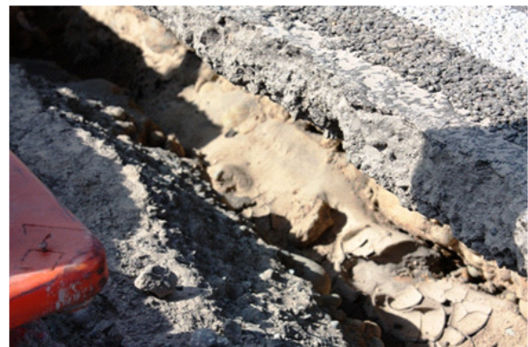
Figure 10. Liquefaction on road 5 South, Santiago-Concepción.
