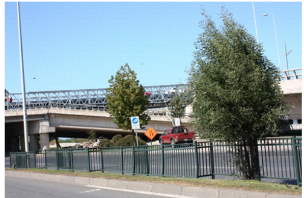
Figure 3. Provisional metal bridge over collapsed section of bridge over Bío Bío river, Concepción.
