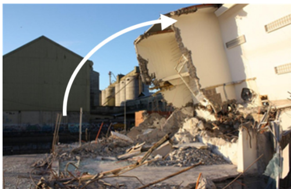
Figure 23. Final tension failure of the front portion of the ground floor, which determined the building's overturn and collapse.
