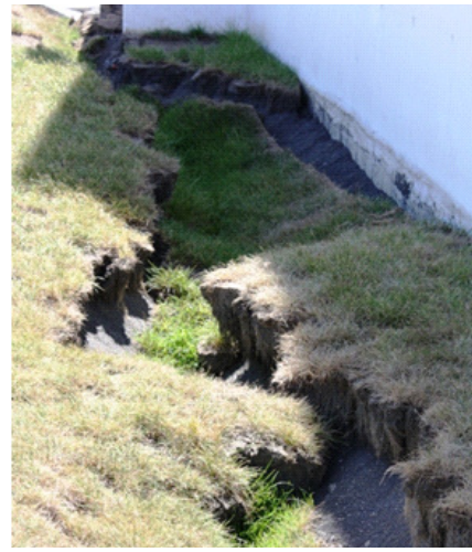
Figure 14. Cracking parallel to the school's constructions, caused by liquefaction. San Pedro La Paz.
