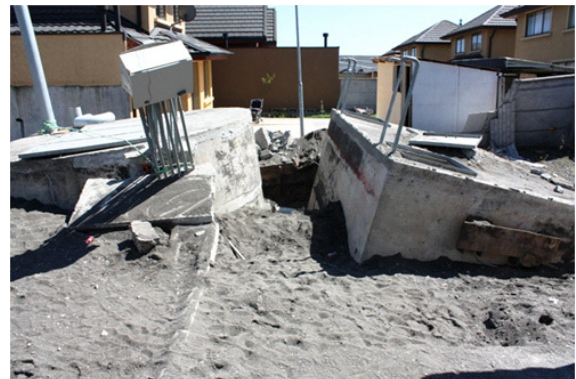
Figure 15. Flotation of boxes of a treatment plant in San Pedro La Paz.
