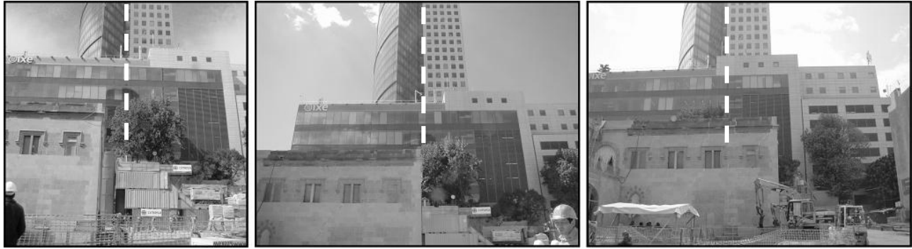
Figure 13. Sequence showing the movement of the house taking as reference one of the edges of Torre Mayor.
