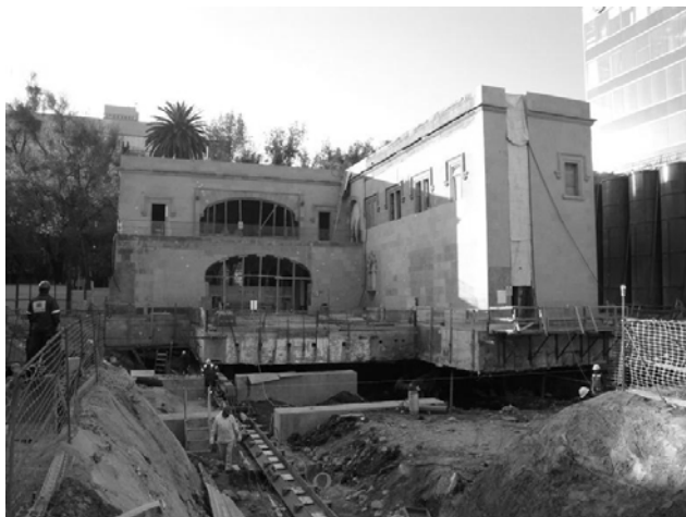
Figure 5. View of the house prior to the movement
