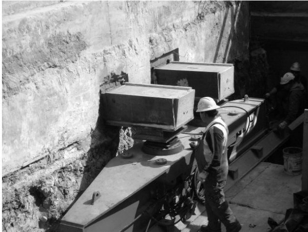
Figure 8. Detail showing the hydraulic jacks (skid shoes) and the brackets embedded in the foundation slab
