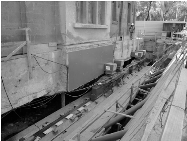
Figure 11. System SKS1000 constituted by modular rails and sliding runners (skid shoes)
