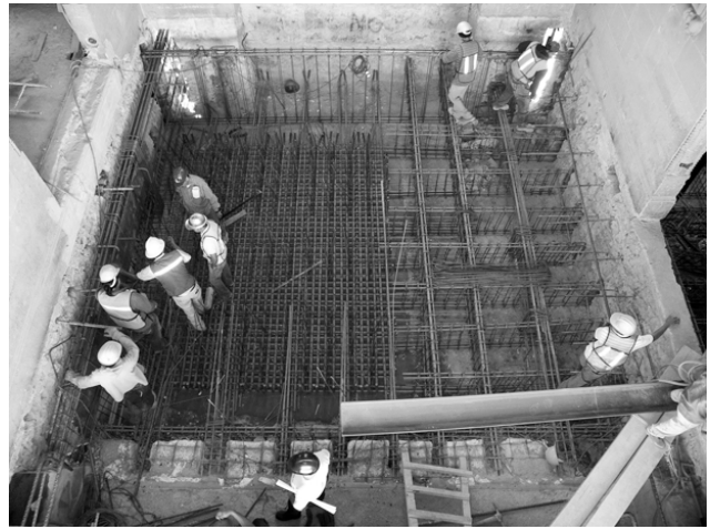
Figure 6. Construction of the ribbed slab for underpinning
