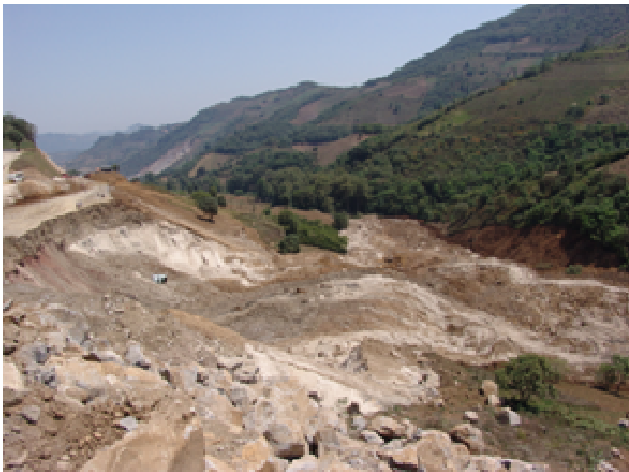
Figure 4. Remnant escarpment of failure (at left) and flow of the failed material toward the river bed (at right)
