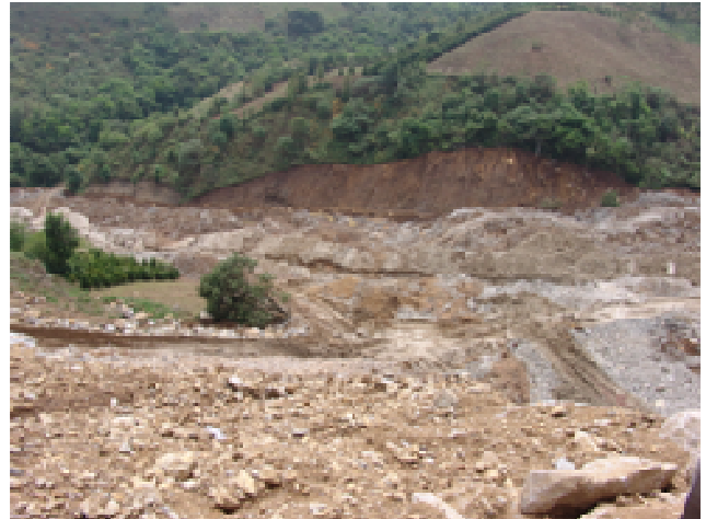
Figure 6. Traces of the splash against the right bank of the failed material that flowed like a fluid
