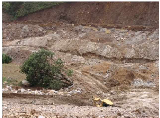
Figure 7. Tree dragged by the failed material
