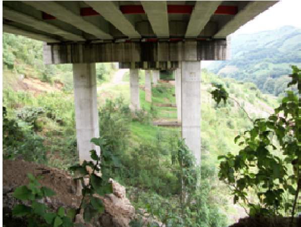
Figure 9. Solution based on a viaduct, applied to the section failed
