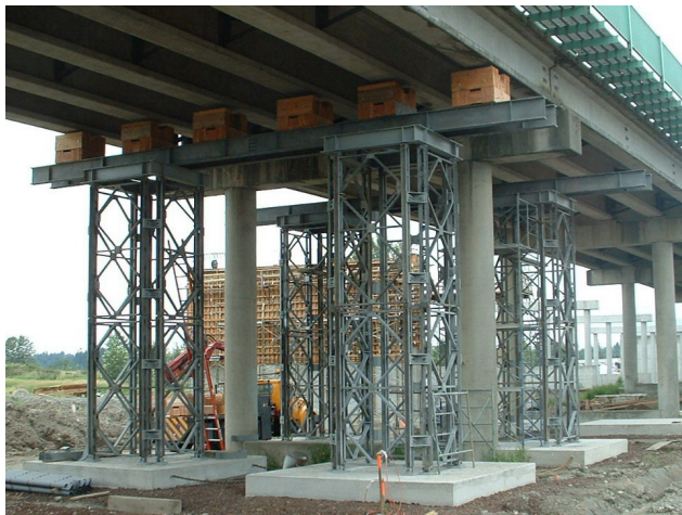
Figure 17. Temporary support towers as constructed
