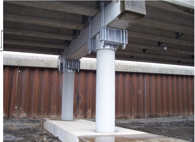
Figure 21. Bent after permanent retrofit (looking west)
