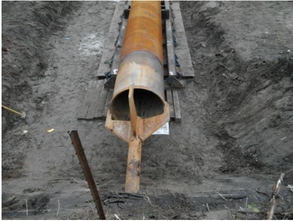
Figure 5. "Spider" attachment connecting 30 inch casing for first Installation to 6 inch pilot string, protruding from embankment.
