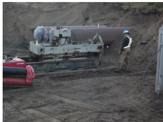
Figure 4. Bore rig preparing to install 6 inch pilot hole beside first two installed pipelines.
