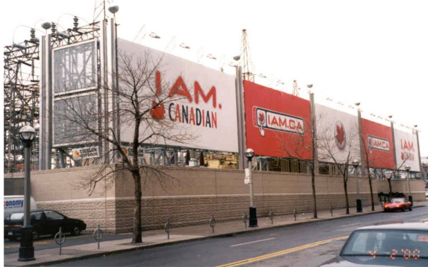
Figure 12. Billboards supported using helical piles
