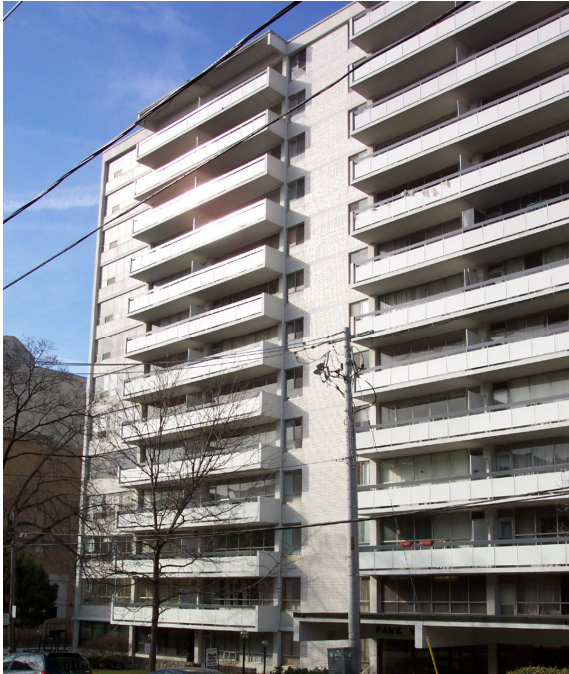
Figure 4. Photograph of 13-storey residential building. After an investigation, petroleum hydrocarbon contamination was found in soils underneath the building, and immediate action was required. Multiple environmental remediation techniques were considered for this project, but in the end a remedial excavation where the soils could be removed safely and treated offsite was deemed the most effective solution in this situation. Traditional underpinning methods were considered, but column loads in excess of 2669 kN and limited head room in the parking garage made these options very expensive and time consuming.
