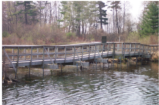
Figure 11. Boardwalk supported using helical piles
