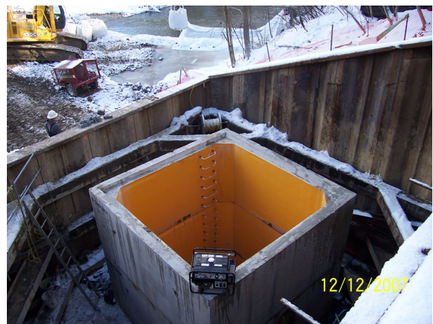
Figure 8. Fox Hollow sanitary trunk sewer manhole
